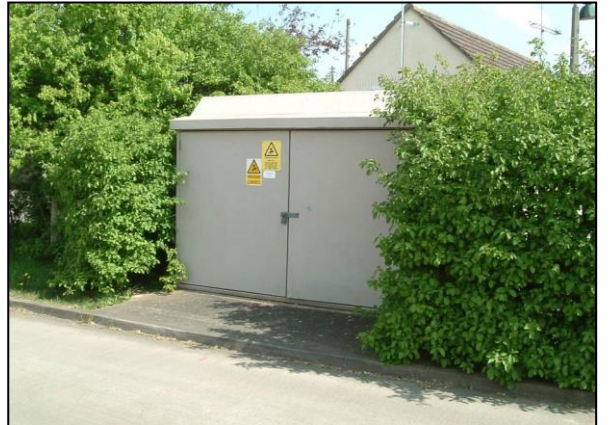
Photograph 4 Distribution Substation
